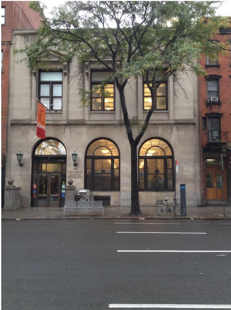
(Image 4) The Columbus Branch of the New York Public Library, 10 th Avenue between 50 th and 51 st Streets, Babb, Cook & Willard, architects (author's photograph).
