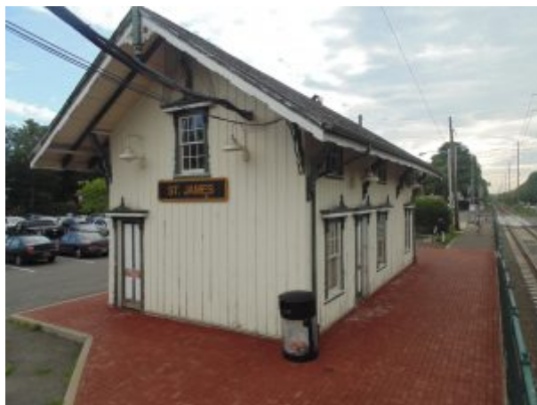
Figure 5. LIRR St. James Station building, built in 1873 (2014: Collection of Derek Stadler)
