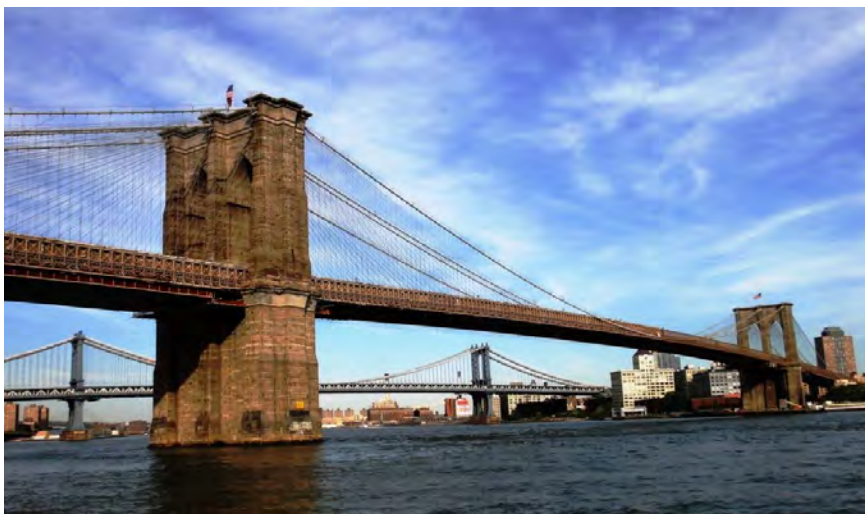
Figure 6. Below the water line the Brooklyn Bridge is faced with rock made of insoluble minerals. Limestone, a more soluble mineral, faces the support above the water line. Image from Ankur Agrawal , CC BY-SA 3.0,
