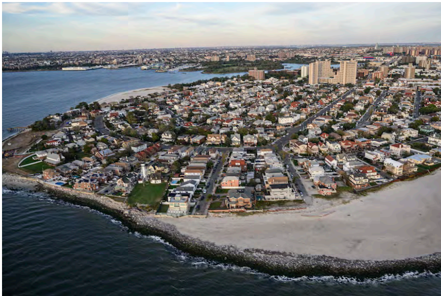
Figure. 1. With houses built right on the coastline, the Rockaways were hit hard by superstorm Sandy in 2012 and are still vulnerable. From van Lohuizen, K. (2018). Rising sea levels and New York City.
