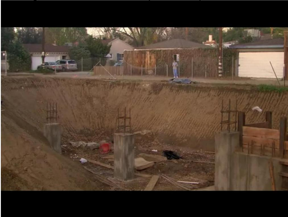
And explain how the steep edges depicted in the picture can be especially dangerous, or how the construction materials in the bottom of the pit could cause extra injuries for someone who falls in.
