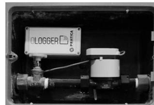
Figure 7. Household flow meter with datalogger deployed
