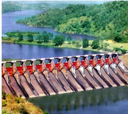
Figure 2. Spillway and chute of the Karnafuli dam in Bangladesh
