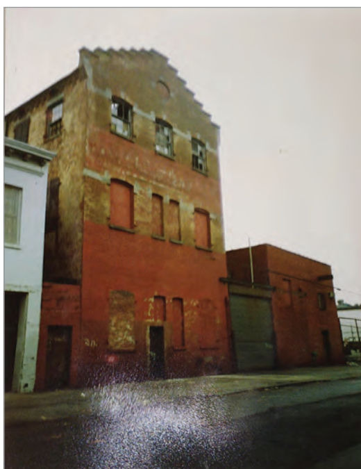
Figure 5: Glare removal seems to depend on lighting conditions and does not always work.
