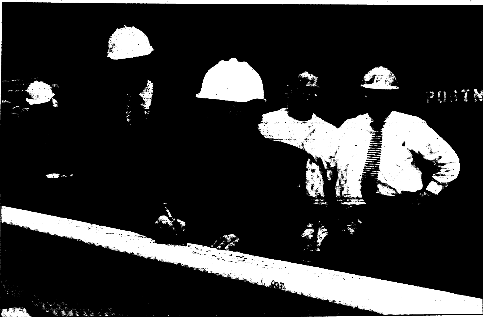
Interim President celebrates on last piece of steel to go on Site B Acting Provost Pickens watches over Interim President Cronholm's shoulder as she autographs the final steel beam to go on the skeletal structure of the Academic Complex, last Thursday, at the Topping Off ceremony. Photograph Courtesy of Baruch College Press Office
