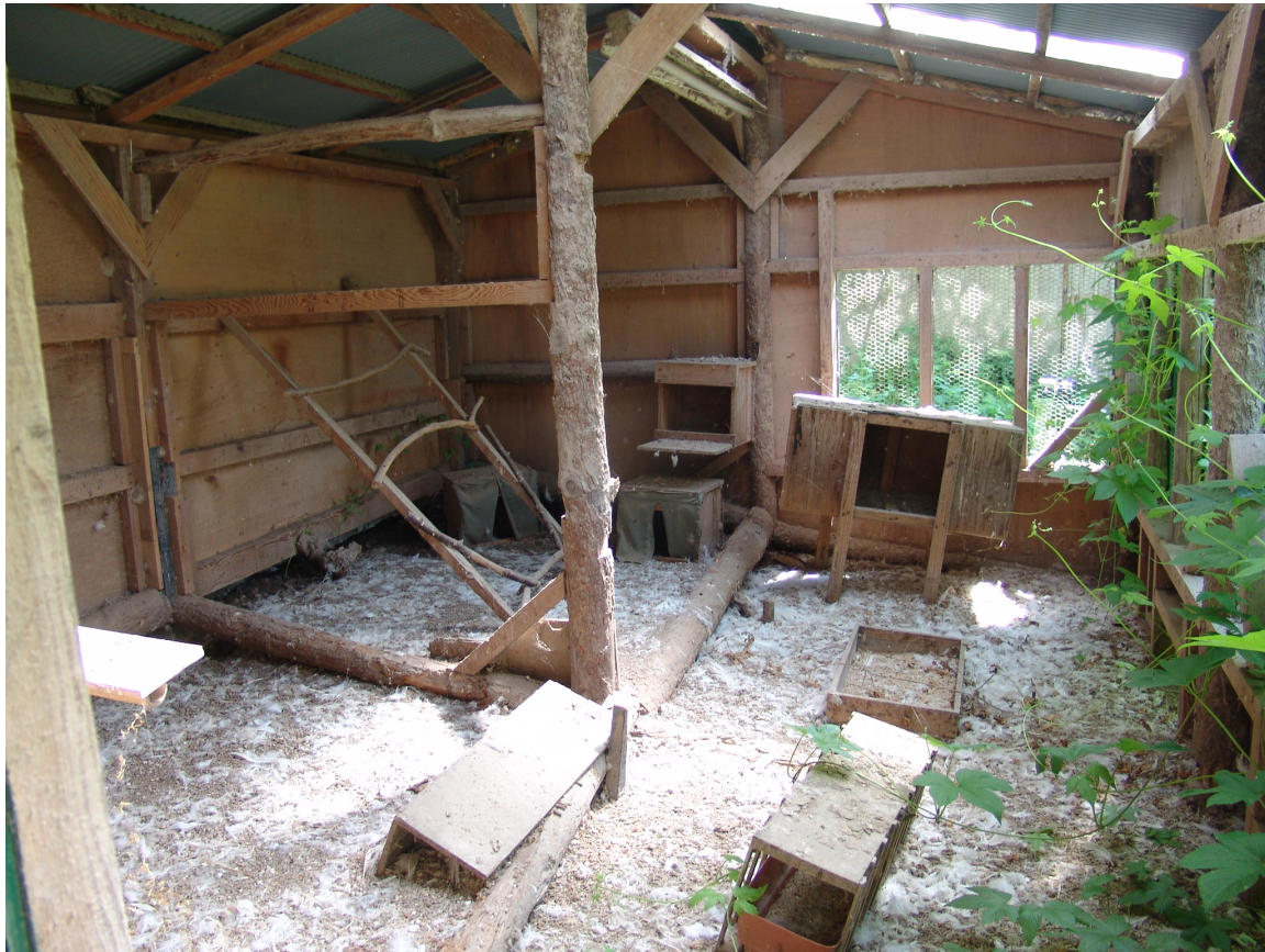
Fig. 15 Interior of a disused chicken coop at Honmura Village, August 2011. The coop is constructed of the same types of materials as the set for Kidnapping above: unfinished wood, processed lumber, and bamboo. Photograph by author.
